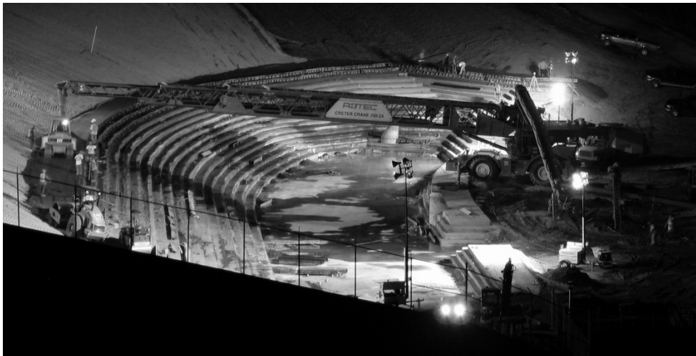
Figure 6. Placement of RCC armouring to embankment dam
